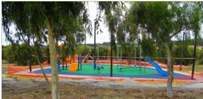
Sussex Bend Playground under construction
