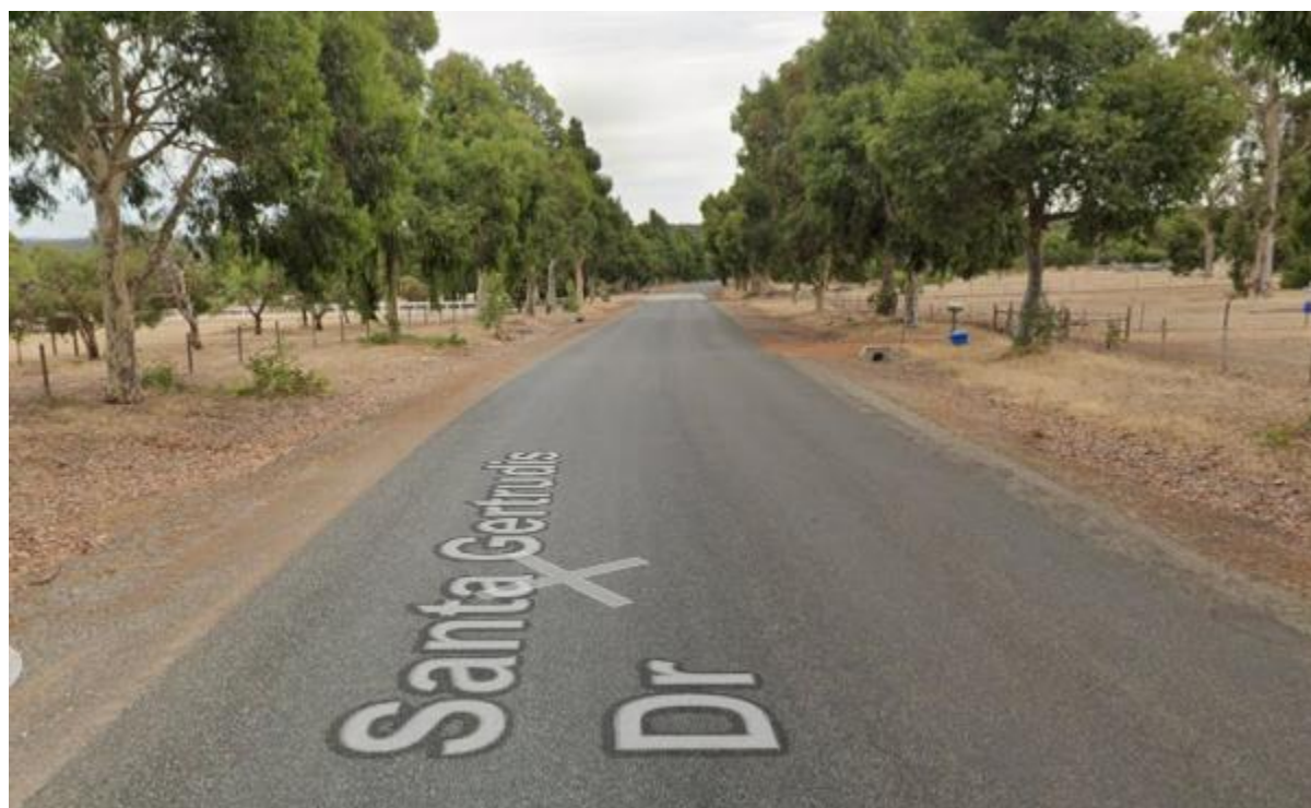
Figure 5 : Typical view of Santa Gertrudis Drive showing drainage swales, culvert crossovers and trees with in the road reserve (Source: Google Maps 2026)
