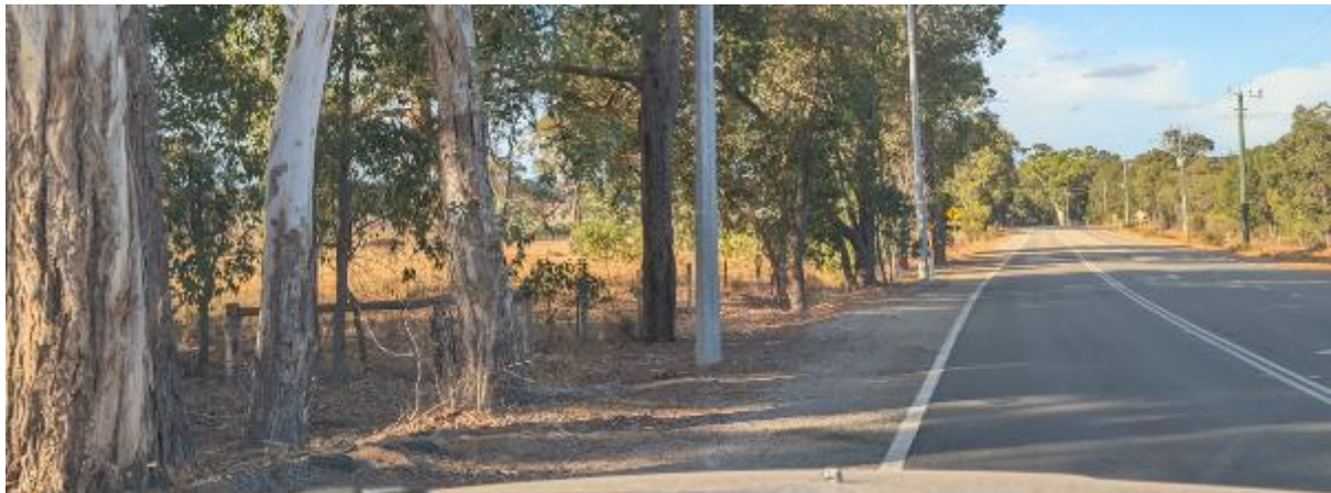
Figure 9 - Section 1 - Muchea East Road (Northern Side)
