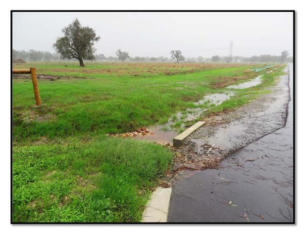
Figure 9 Concept drainage showing storm runoff from roads to an adjoining grassed swale drain, in the same manner that is proposed for Lot 7. Notice the potential for infiltration within the drain.
