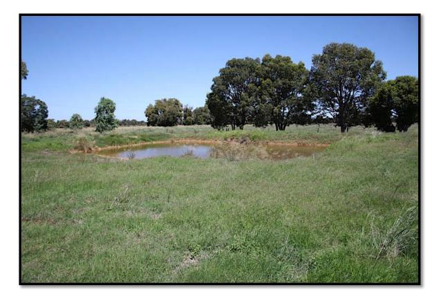
Figure 11 Existing water detention basin on Lot 3. Infiltration is through the bund wall towards the trees. Note the pasture that is providing filtration and slowing of the surface water flows.
