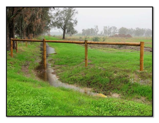
Figure 10 Concept grassed swale drain during storm event, that allows for infiltration, slowing of the flows and is adjacent to tree belts as proposed for the hardstand on Lot 7.
