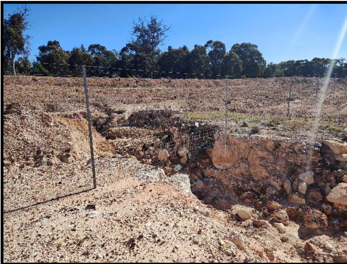
Photo 4: Stormwater channel flowing from Lot 9001 to the Shire's Muchea landfill site.
