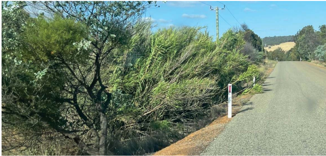
Photograph 5 – Example of steep embankment/ drop-off close to edge of 110 km/h road
