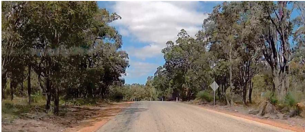
Dashcam Photograph 1 – Driving east at SLK 1.68: crest and left bend restricts sight distance to approx 130 m – required SSD at 110 km/h: 278 m
