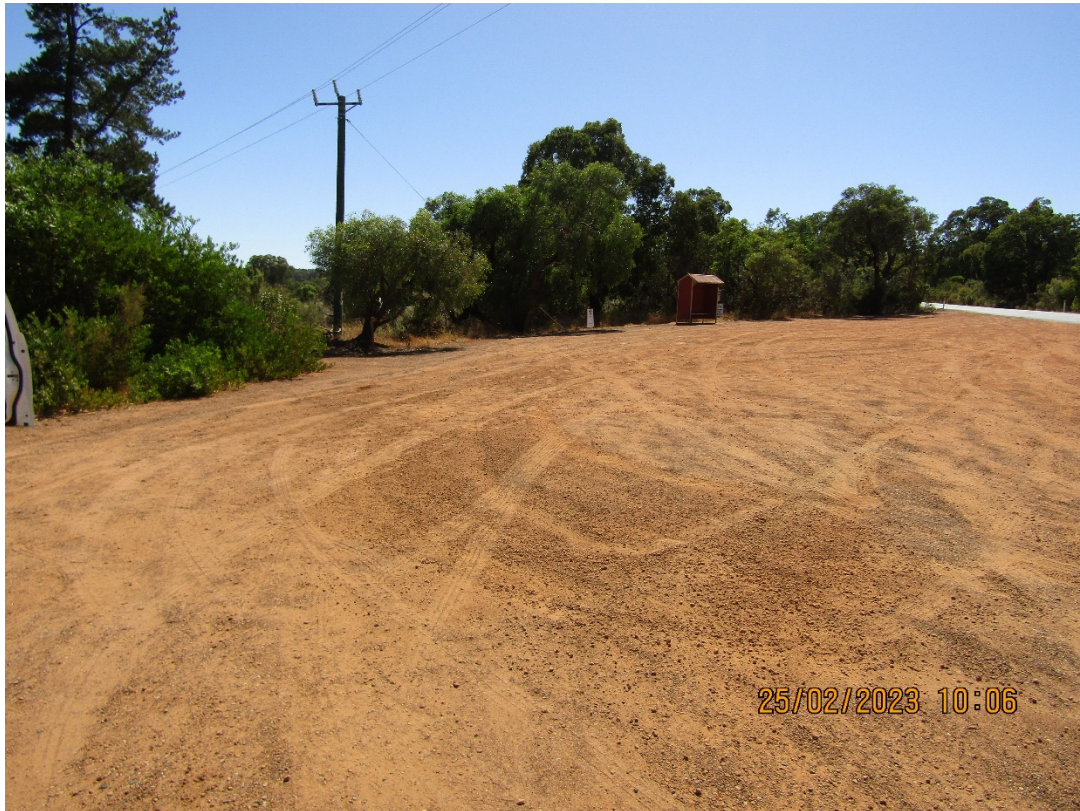
Blue Plains Road and Great Northern Highway Intersection
