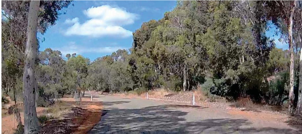
Dashcam Photograph 4 – Driving east at SLK 4.95: left bend restricts sight distance to approx 80 m – required SSD at 60 km/h advisory speed: 98 m
