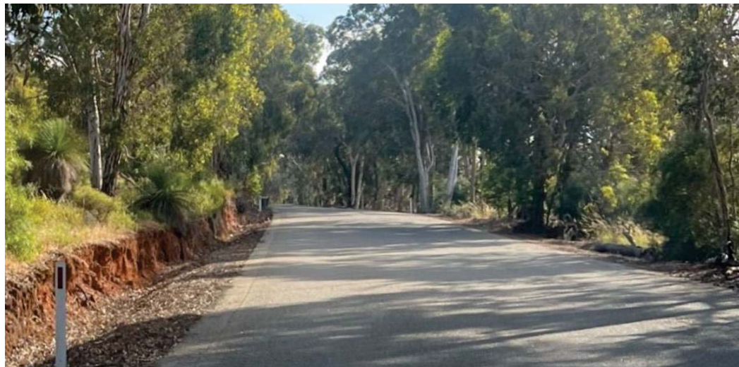
Photograph 6 – Example of steep embankment (cut) close to edge of 110 km/h road
