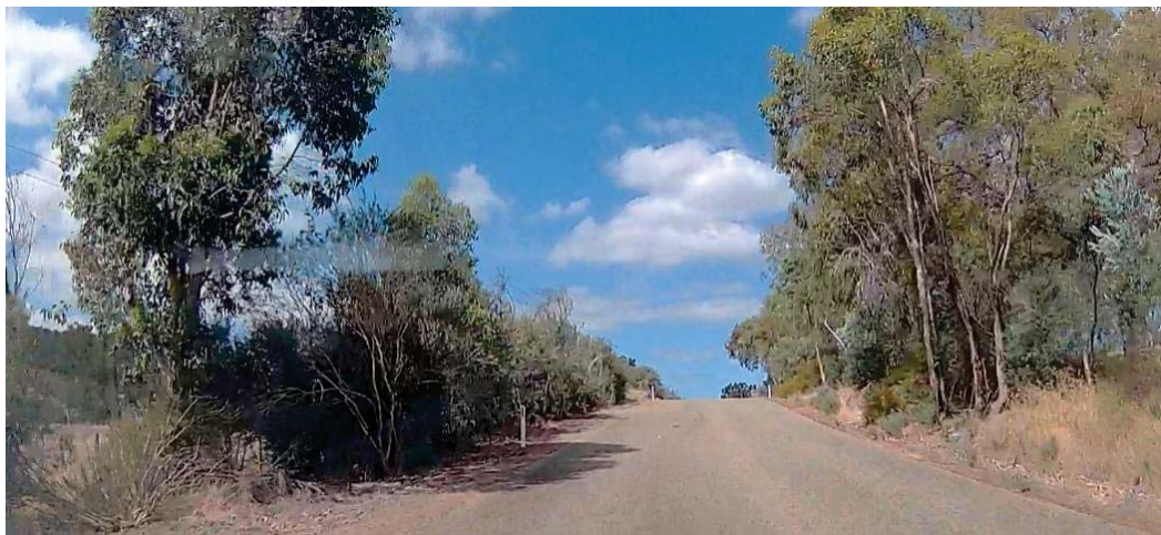
Dashcam Photograph 5 – Driving east at SLK 5.33: crest restricts sight distance to approx 80 m – required SSD at 110 km/h: 278 m
