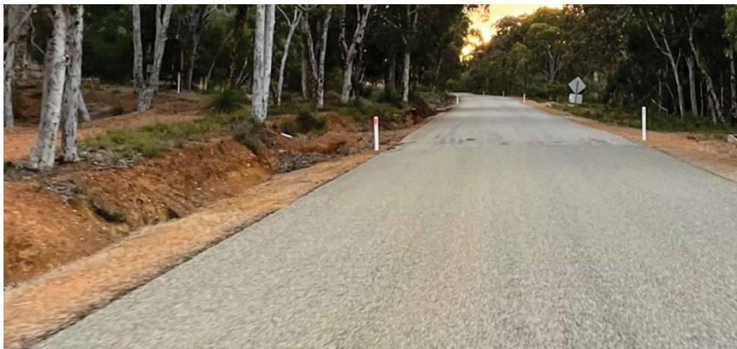
Photograph 7 – Example of open drain close to edge of 110 km/h road
