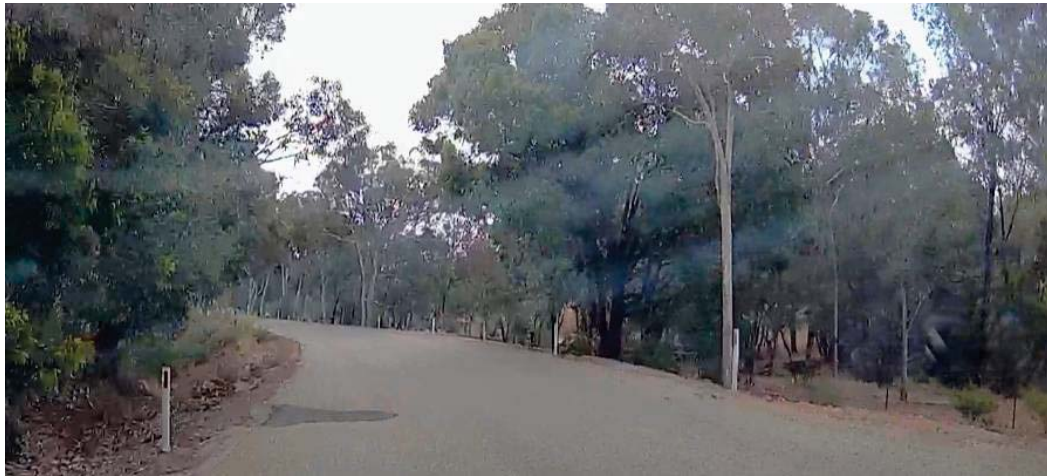
Dashcam Photograph 7 – Driving west at SLK 4.69 to SLK 4.62: left bend restricts sight distance to approx 80 m – required SSD at 110 km/h: 278 m
