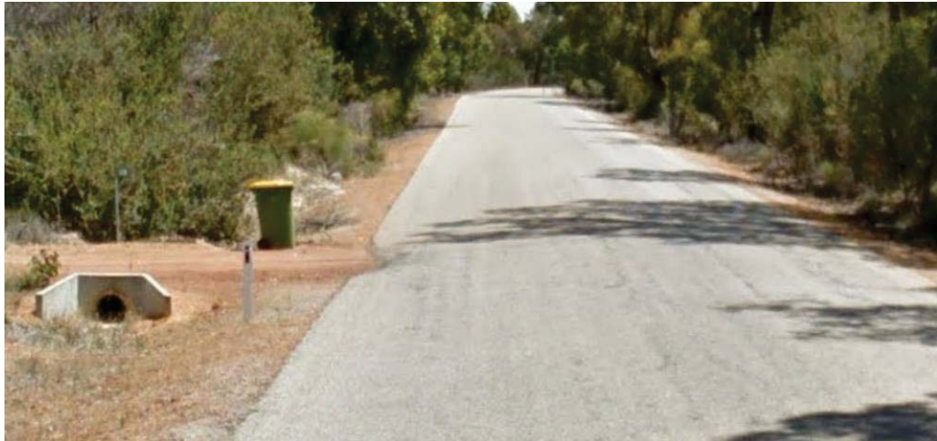
Photograph 3 – Example of culvert structure within 2.3 m of 110 km/h road
