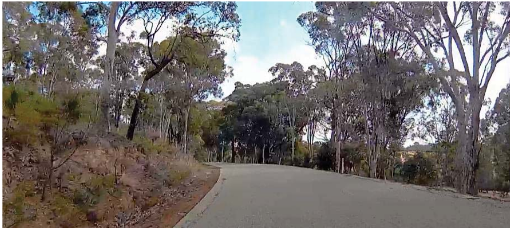
Dashcam Photograph 8 – Driving west at SLK 4.15: left bend restricts sight distance to approx 90 m – required SSD at 110 km/h: 278 m
