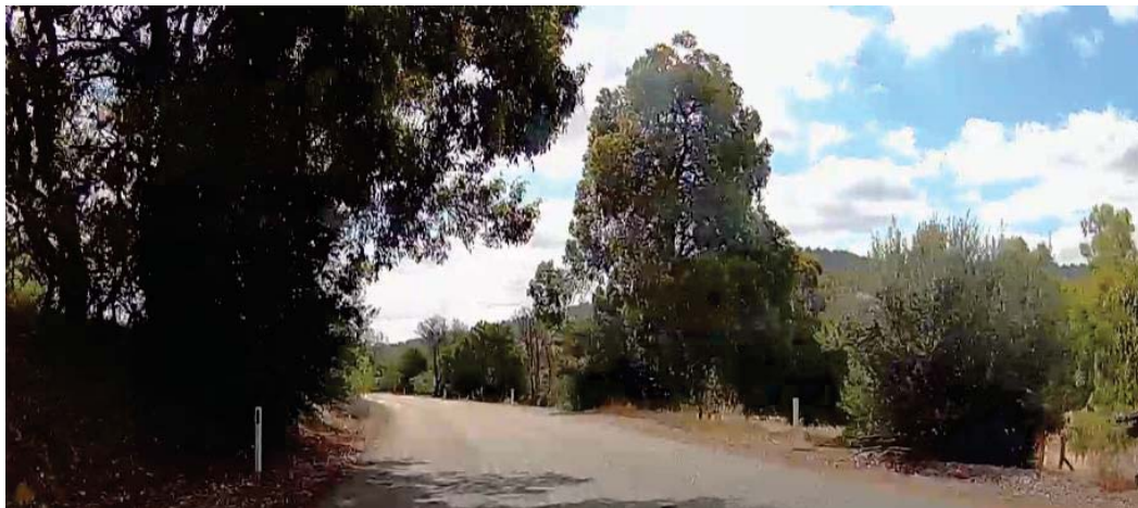
Dashcam Photograph 6 – Driving west at SLK 6.86 to SLK 6.64: left bend restricts sight distance to approx 100 m – required SSD at 110 km/h: 278 m
