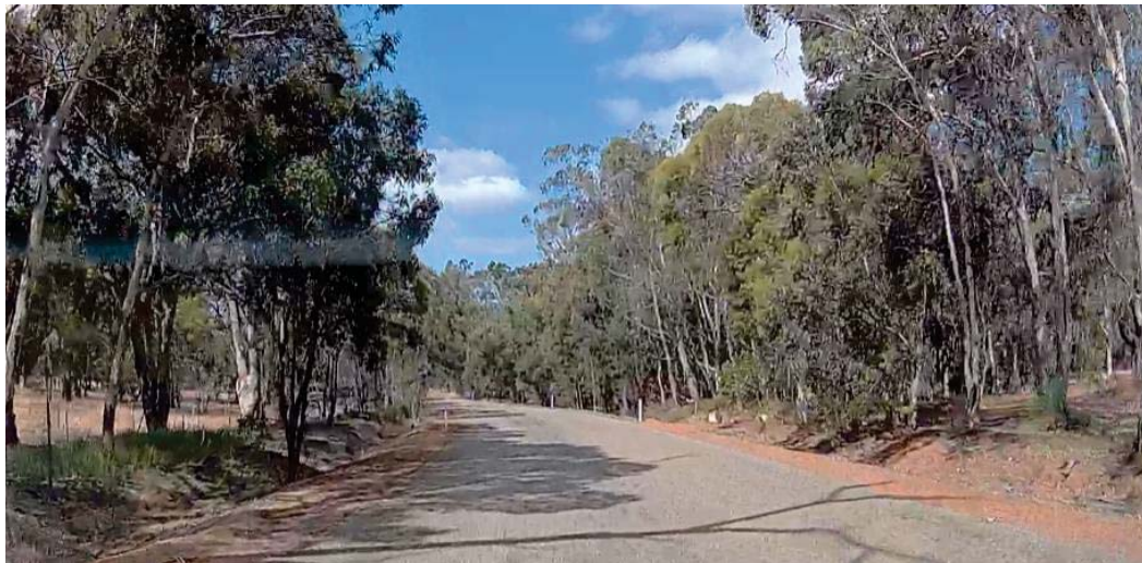
Dashcam Photograph 2 – Driving east at SLK 3.09: left bend restricts sight distance to approx 140 m – required SSD at 60 km/h advisory speed: 98 m
