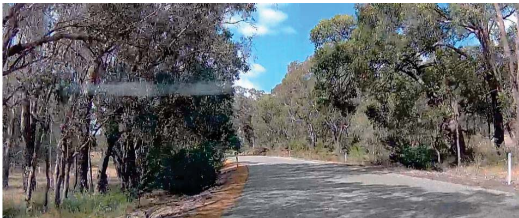
Dashcam Photograph 3 – Driving east at SLK 3.45: left bend restricts sight distance to approx 60 m – required SSD at 110 km/h: 278 m
