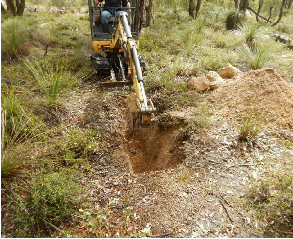
Photo 3. Excavating Test Pit at Test Location 01 (TP1)
