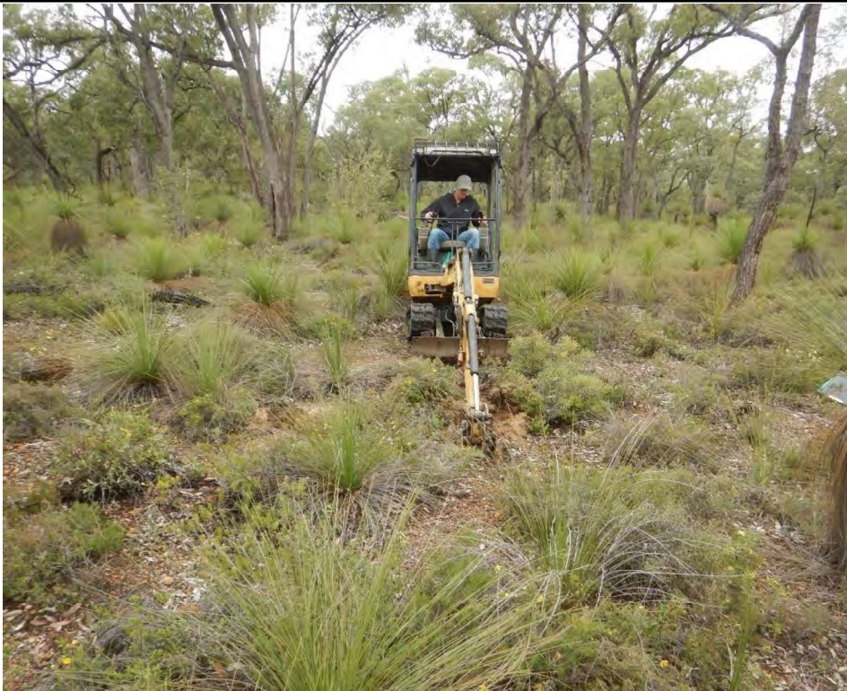
Photo 8. Excavating Test Pit at Test Location 06 (TP6)
