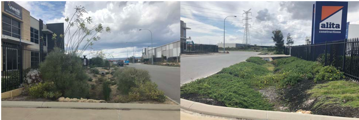
VEGETATED STORMWATER SWALE CONCEPT
