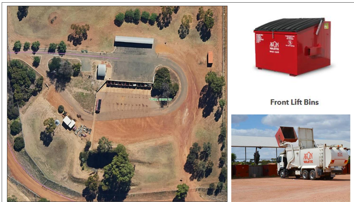
Figure 5.1 Example of a transfer station utilising a front lift bin system, servicing truck and bin type
