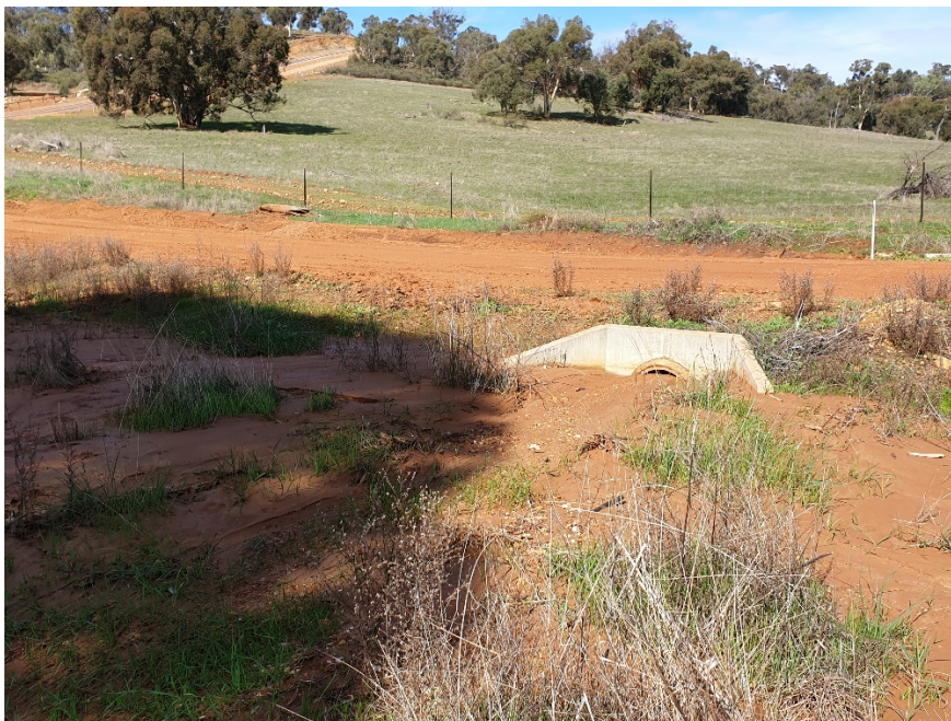
Blocked drain. Kay Road: 27 th July 2019
