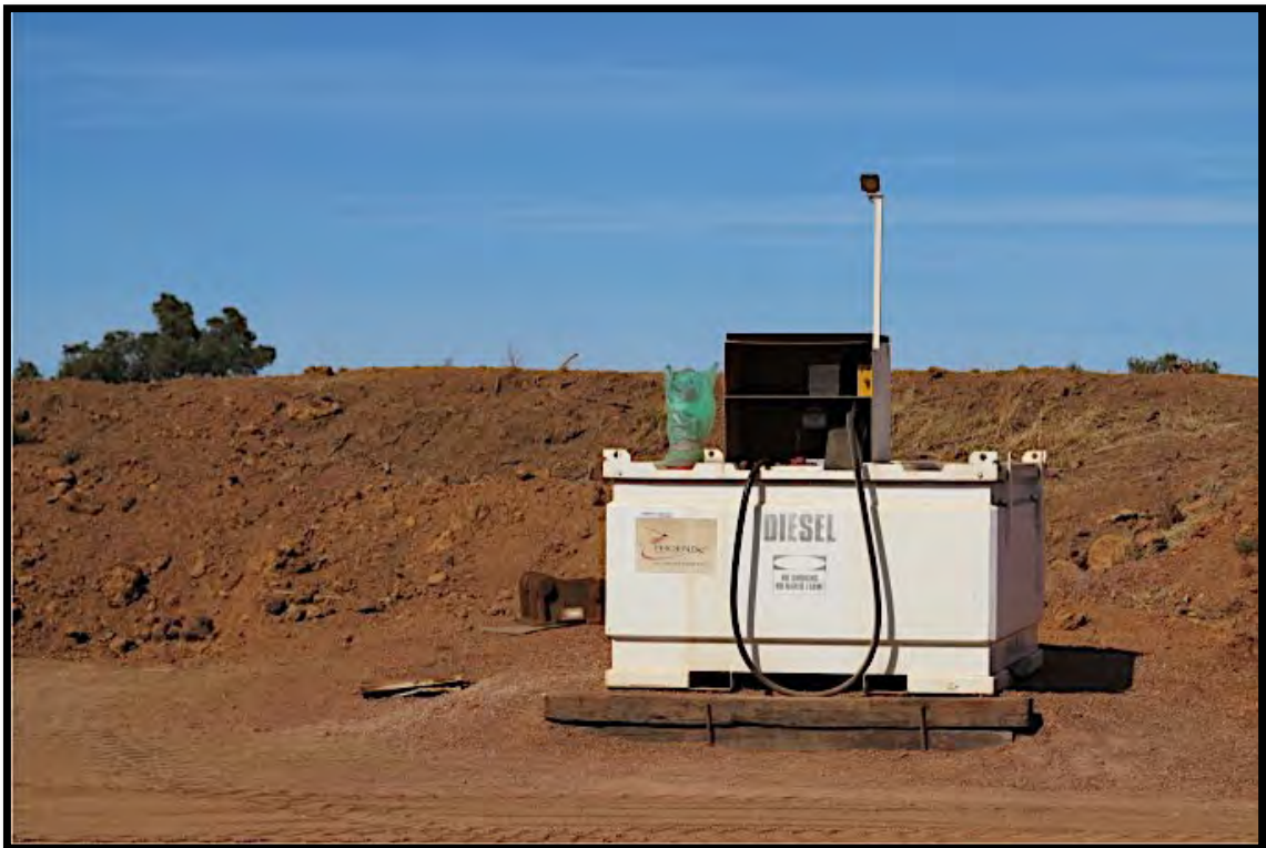
Figure 10: Approved double skinned temporary storage
