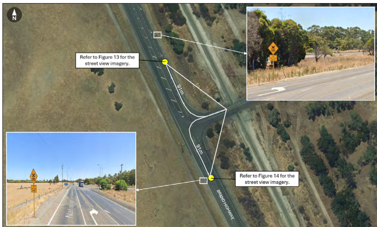
Figure 12 Stopping Sight Distances and Warning Signage at Brand Highway and Railway Crossing
