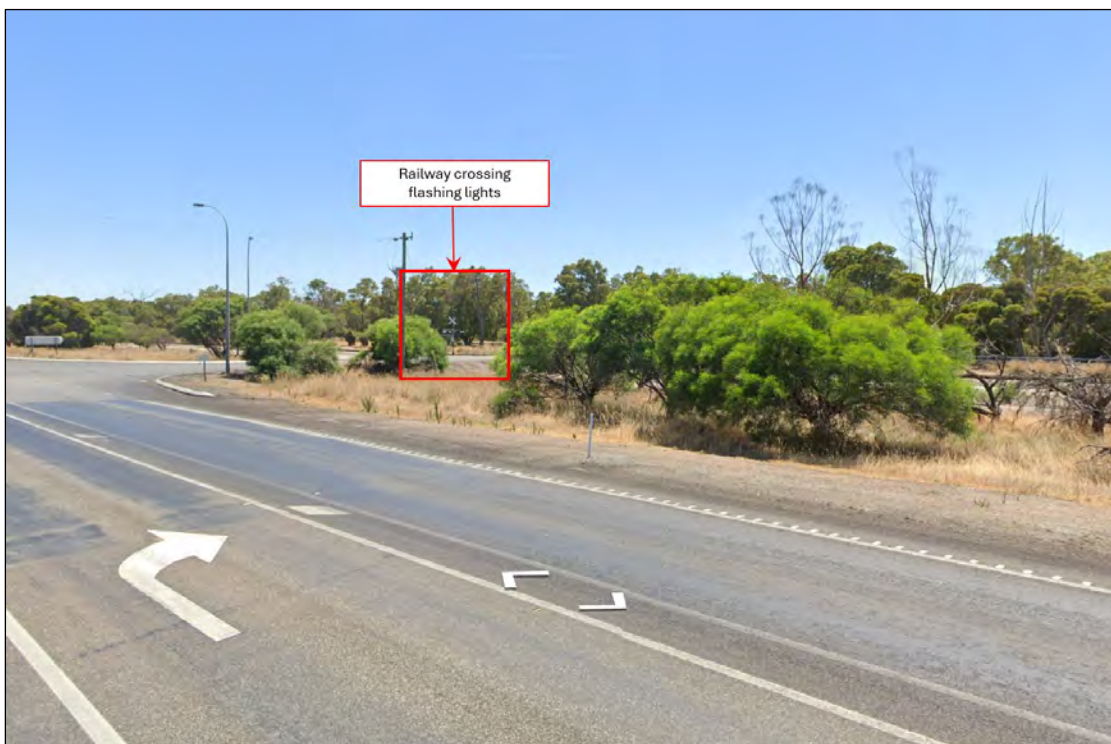
Figure 14 Driver's View of the Flashing Lights at 91m Stopping Sight Distance (at the south approach of Brand Highway)
