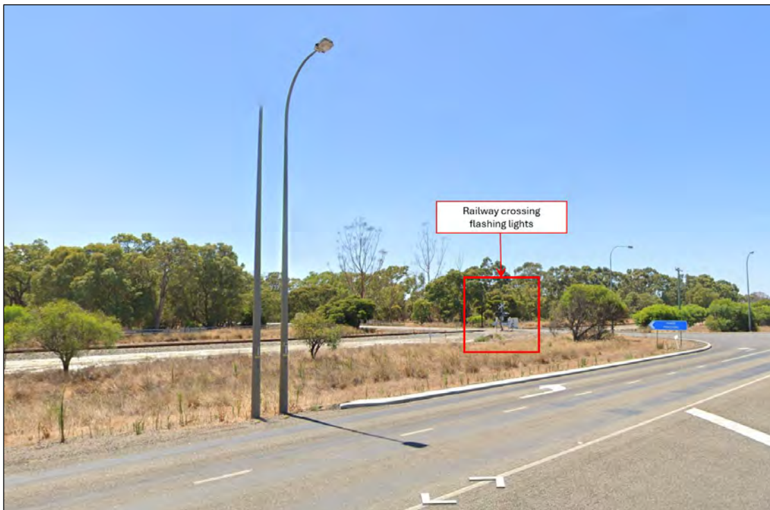
Figure 13 Driver's View of the Flashing Lights at 91m Stopping Sight Distance (at the north approach of Brand Highway)
