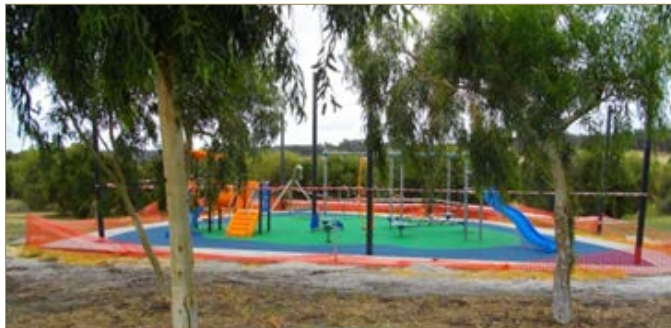
Sussex Bend Playground under construction
