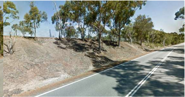
3 Wandena Rd looking north-west towards Lot 202
