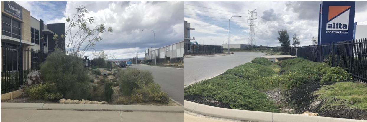
VEGETATED STORMWATER SWALE CONCEPT
