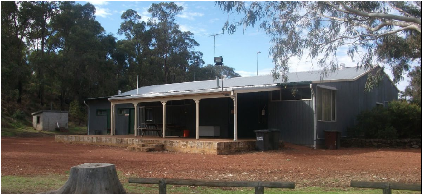
PIC 1: CURRENT LOWER CHITTERING HALL
